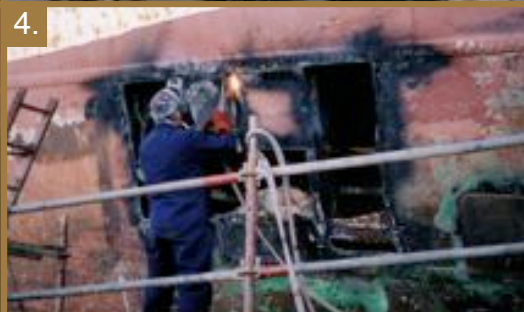
4. Welder cuts through the bow of Harmony II.
